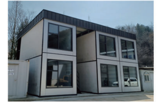
② Goesan Dormitory
